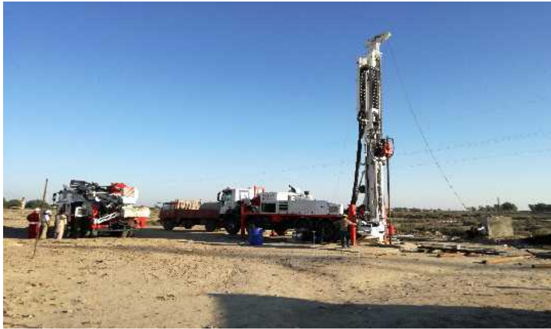
Fig 04: Two Newly Purchased Multipurpose Drilling Rig
